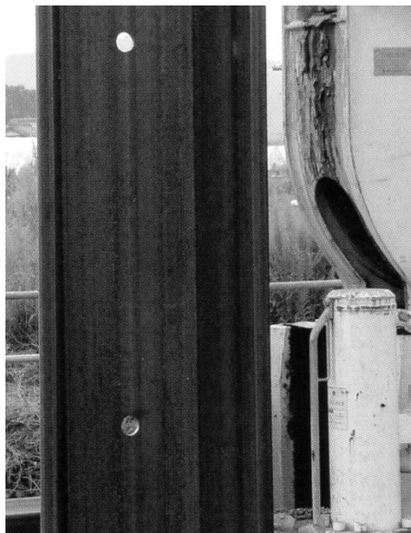
図-4.0.1 透水性鋼矢板
