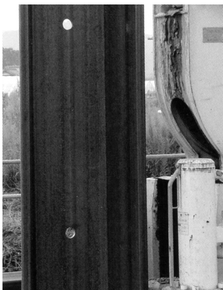
図-4.0.1 透水性鋼矢板
